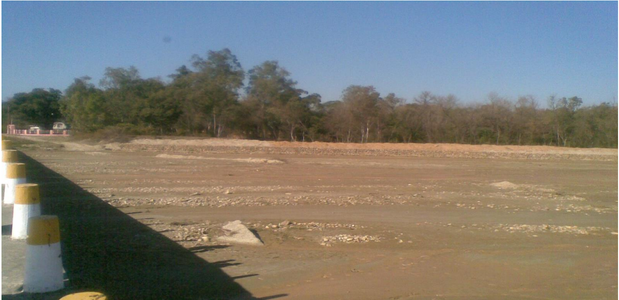
Figure 7.7: A view of Uttar Behni area showing human efforts to check encroachment by the river Devak. Note the embankment constructed on the left bank of the river
