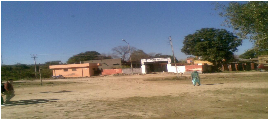
Figure 7.8: A view showing infrastructural development in Purmandal area
